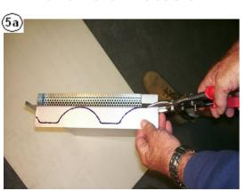
5. Trim vent along texta mark with tin snips, when this is trimmed it will fit the profile of your roof and will also leave a flap of metal to the right hand side of the vent which when fixed in the roof will fit under the tile at the right hand side of the vent. Be sure not to cut too much material away.
