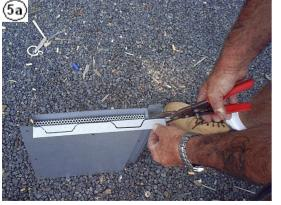
5. Trim vent along texta mark with tin snips, when this is trimmed it will fit the profile of your roof and will also leave a flap of metal to the right hand side of the vent which when fixed in the roof will fit under the tile at the right hand side of the vent. Be sure not to cut too much material away.
