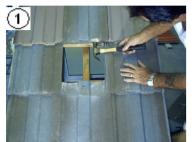
**2A.** Straight bonded roof:-Knock tile lugs off bottom of tile in the course above to allow the tile to sit flush with the vent.
