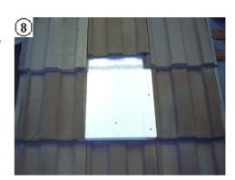
**9.** Pull the tile/s back into position, smooth the silicon out to close all gaps between vent and tile/s (*Be careful not to block out any water courses*). Finally, run a bead of silicon down both sides of the vent attaching the tiles to the vent. The water courses above vent may also be silicon sealed if preferred.
