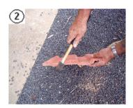
To carry out this step tiles may be left in the roof or removed if possible. However if you prefer you can cut the lugs off using an angle grinder, this way you can grind the lugs completely flat.
